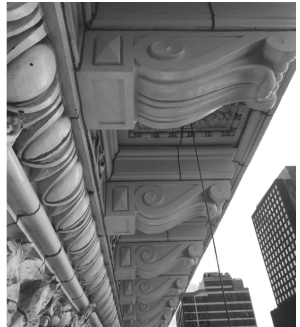
Completed replacement of scroll brackets
