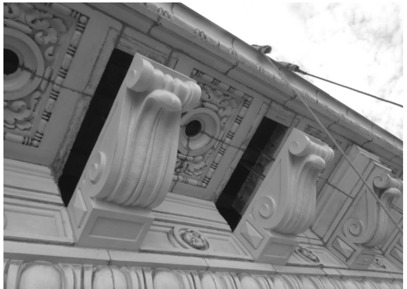
New GFRC scroll brackets being installed
