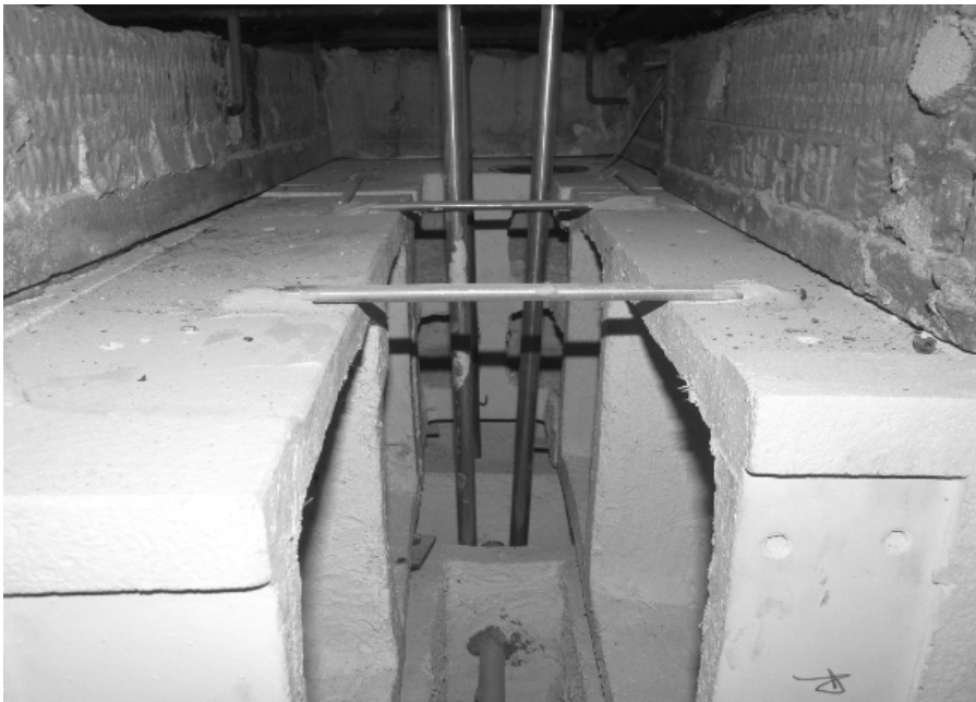
New GFRC scroll brackets with stainless steel 'J' hooks'
