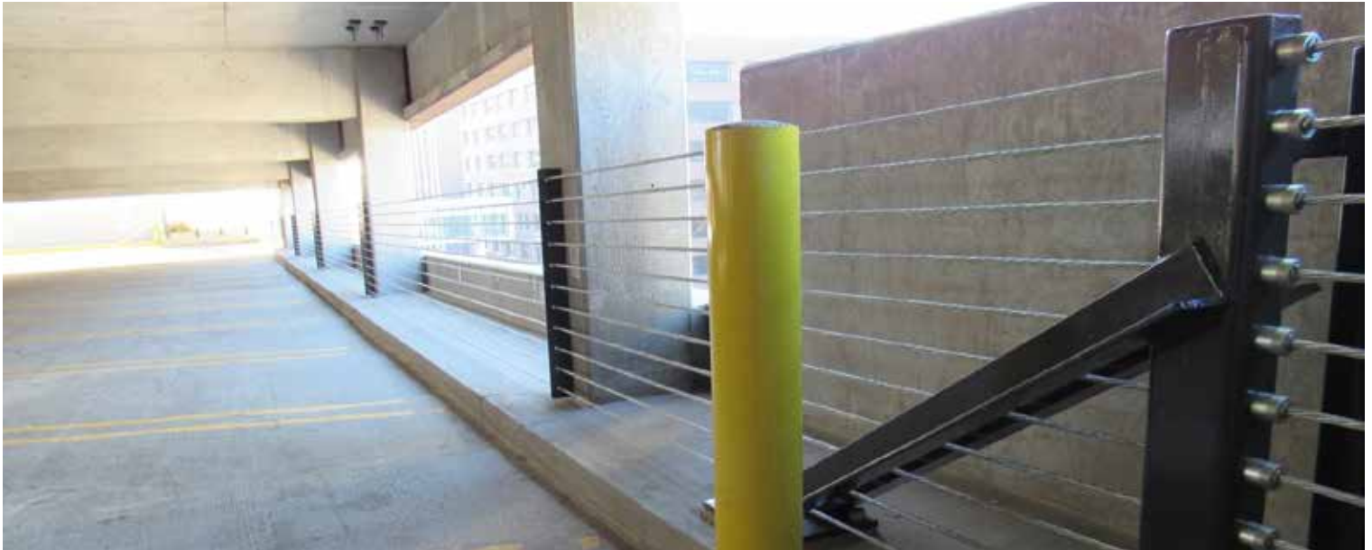
Fig. 4 Typical new vehicle barrier cable installation
