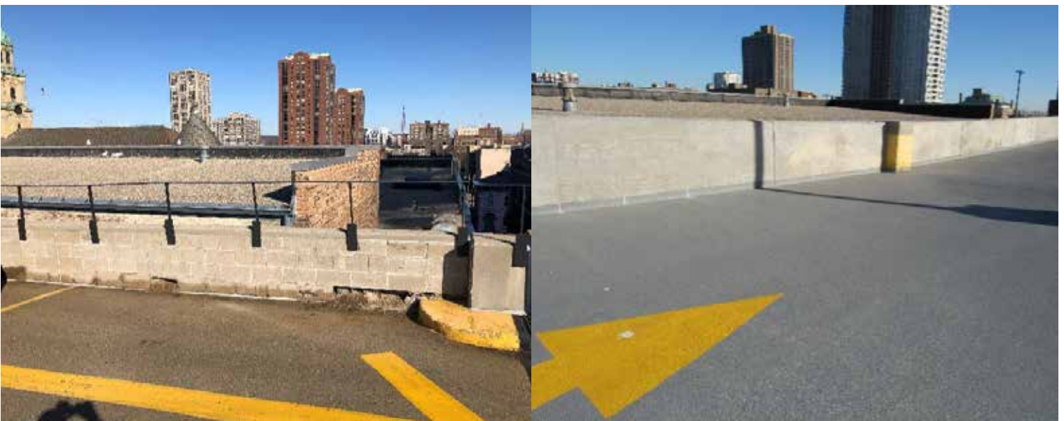
Fig. 3 Before and After Bumper Wall Repair
