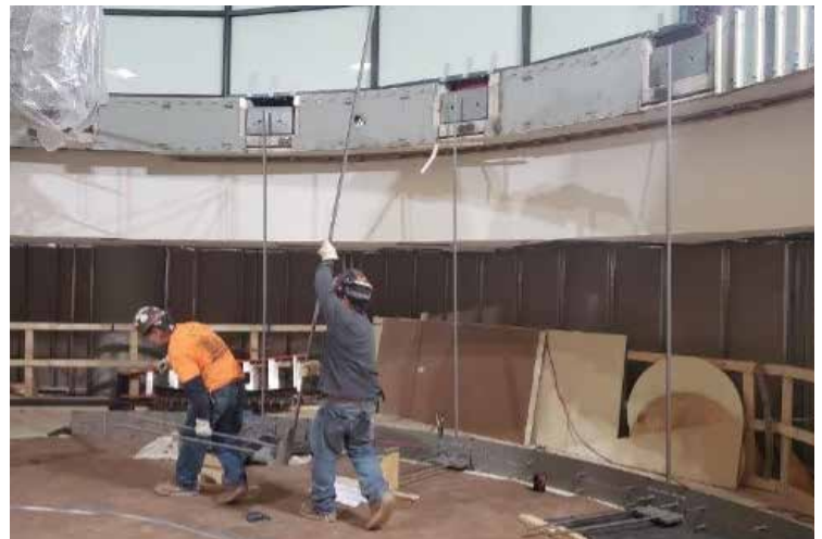
Fig. 3 - Hanger Rod Installation
