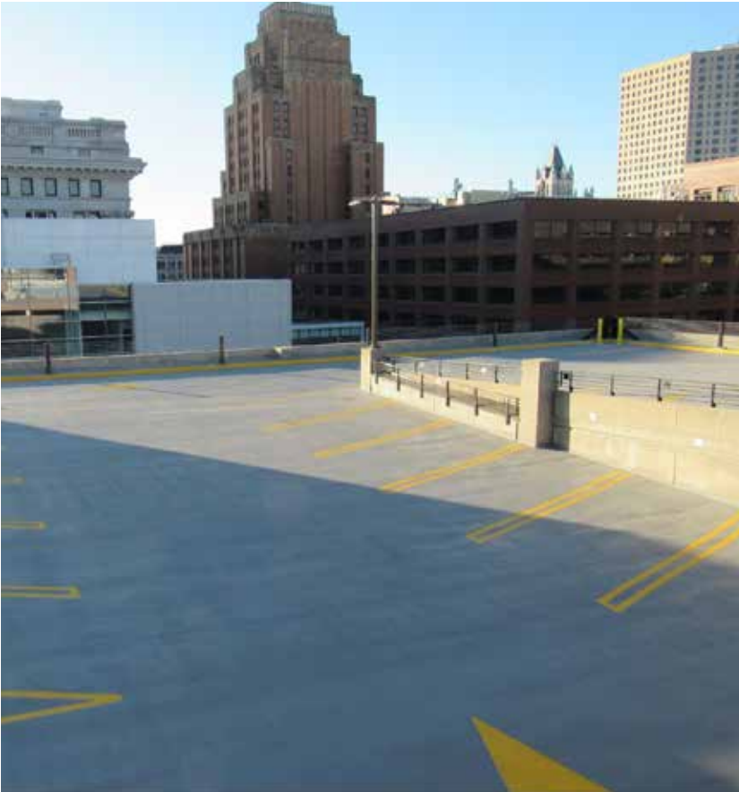
Fig.1 Completed roof level with new Kelmar traffic topping and barrier cables
