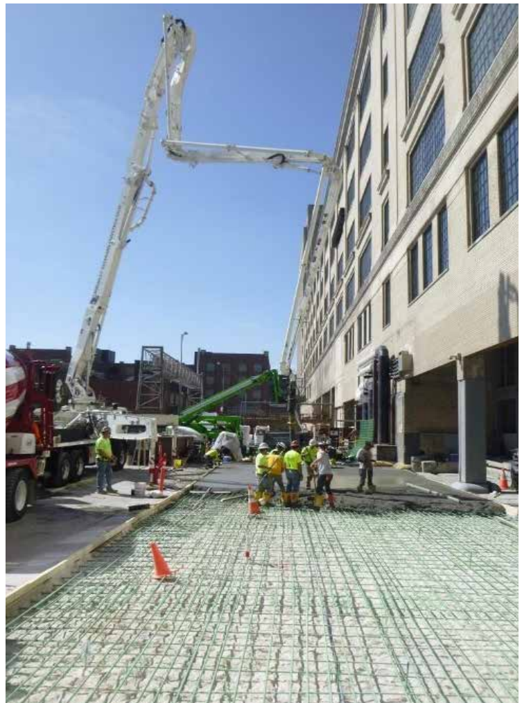
Figure 4. Topside structural slab repair at northeast plaza
