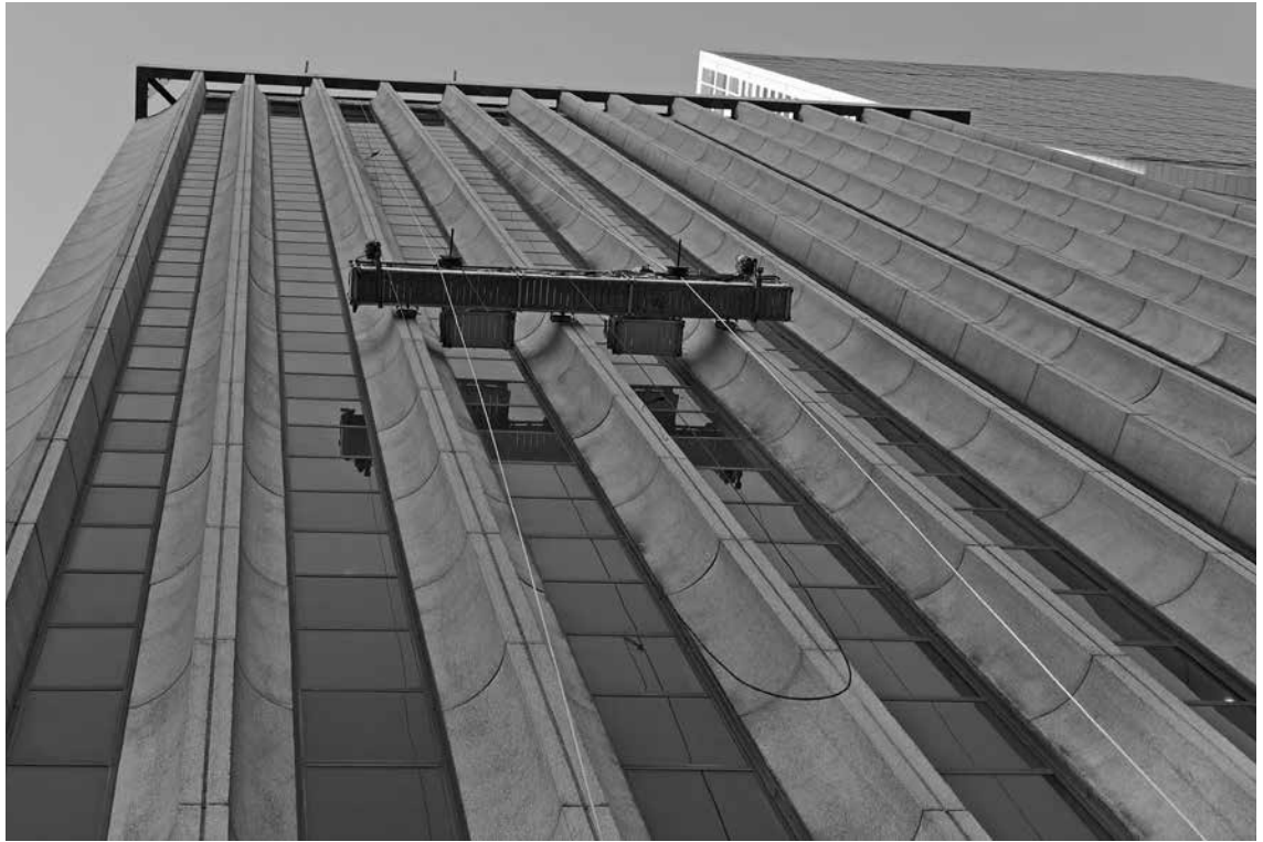
Figure 3: Porch brackets provide access on facades with fins and other architectural features
