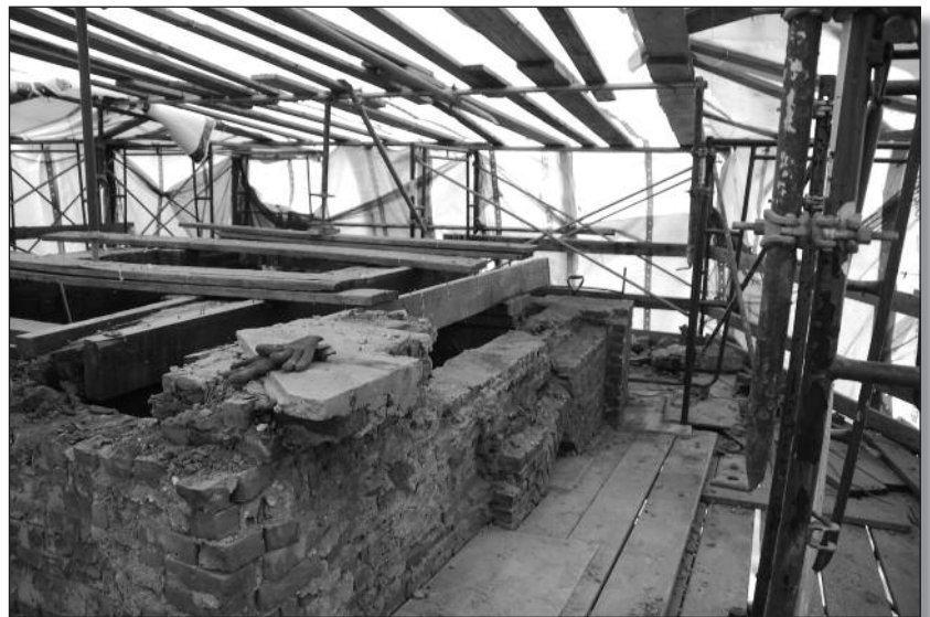
Structural evaluation and repair (Photo courtesy of Acheson Doyle Partners)
